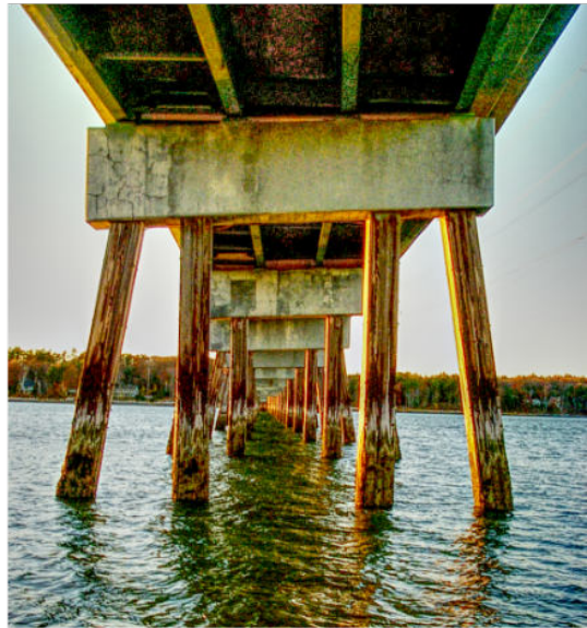
The bridge to Cousin’s Island, Yarmouth, Maine.
