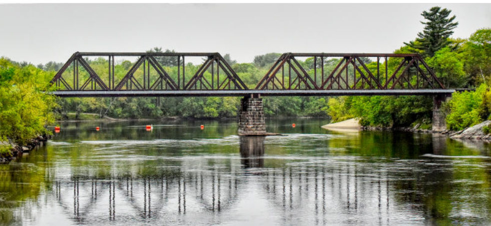
This bridge over the Androscoggin River once had another deck for trains.
