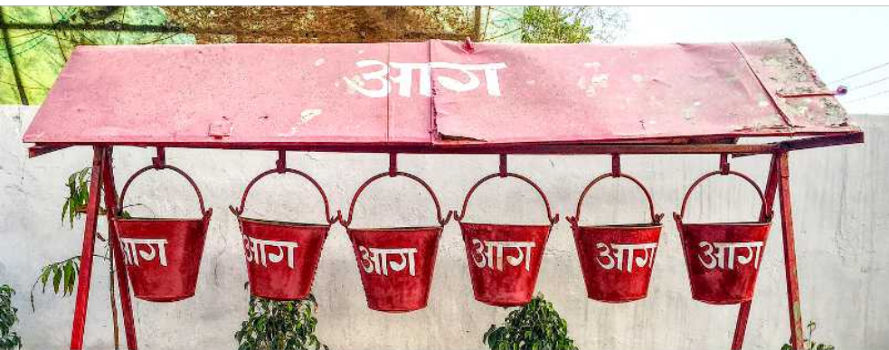
Required at gas stations, like this one in Churu, India, sand can help extinguish fires.
