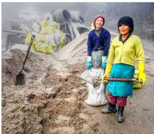
Repairing the road up to Darjeeling.
